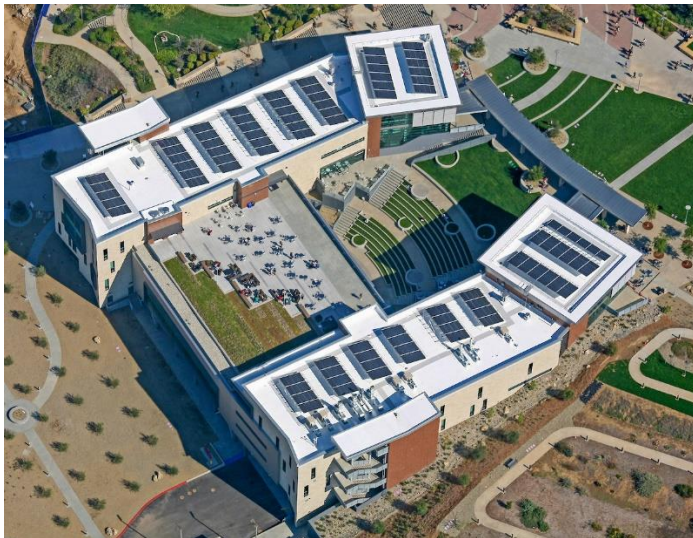
Figure 7. Green Roof at CSU San Marcos
